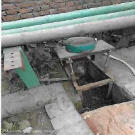
Fig.7: Backwash Effluent Bye-pass
