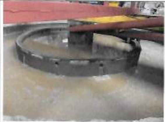
Photo 6: Overflow tank cum storage for recycling
