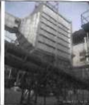
Photo 18: ESP and Stack
