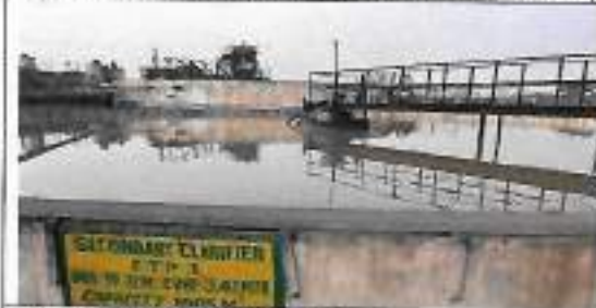
Fig.5: Secondary Clarifier
