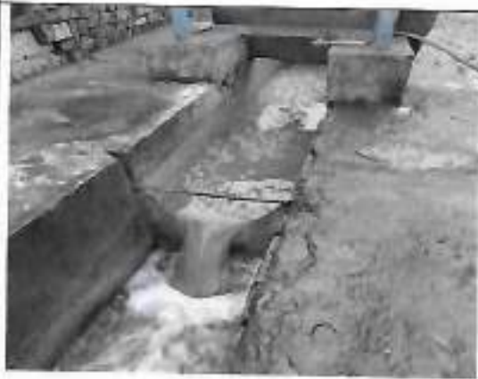
ETP final outlet discharge line (after tertiary treatment units)
