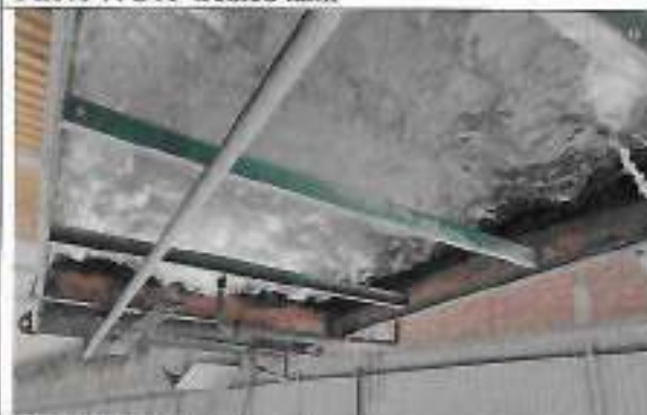
Photo 9: STP Aeration tank
