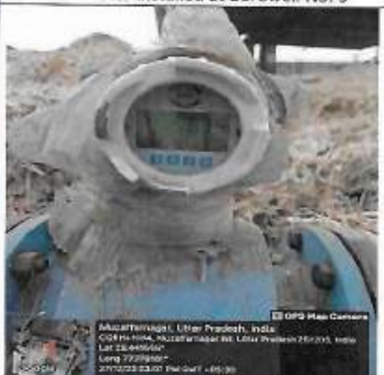
Flow meter installed at effluent recycling line
