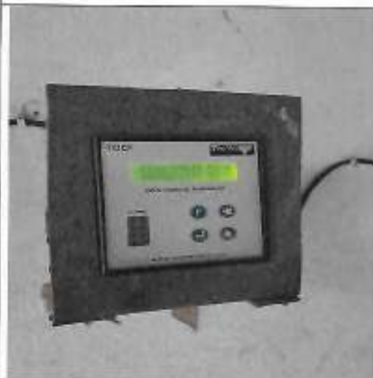
Flow meter installed at ETP Inlet
