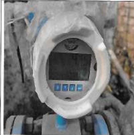
Flow meter installed at ETP Inlet
