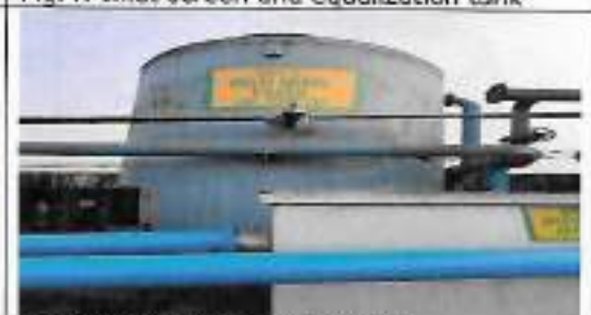
Fig.6: Multi Grade Filter (MGF)
