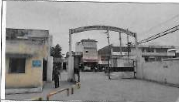
Photo 1: Unit's Entrance Gate
