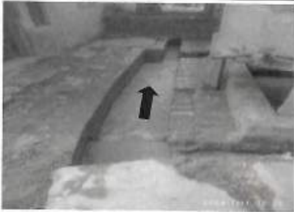
ETP inlet channel
