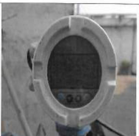
Flow meter installed at effluent recycling line
